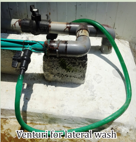
Acidified water being pumped through venturi
